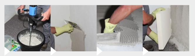
Adhesive SK is mixed with 5.2 liters of water using a slowly rotating electrical mixer into a homogenous, lump free consistency.
