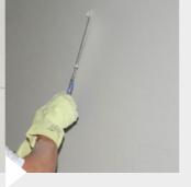
In normal room conditions and with plastered with a layer of KÖSTER good air circulation the surface can be decorated after 24 hours with breathable materials.
