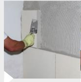
A bead of KÖSTER Hydrosilicate Adhesive SK is applied along edges of the boards to make sure surface can be sanded smooth. that the joints are fully filled.
