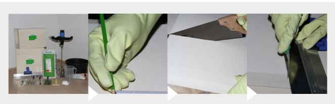
Old wall coverings and bond inhibiting substances such as wallpaper, gypsum residues, paint, or insulation must be completely removed. Absorbent substrates are primed with KÖSTER Polysil TG 500. Irregularities and holes in the surface smaller than 5 mm can be closed with KÖSTER Hydrosilicate Adhesive SK. Larger surface defects can be repaired using KÖSTER Repair Mortar.
