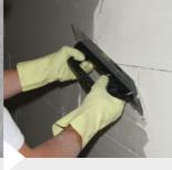
Subsequently the whole area is Hydrosilicate Adhesive SK in a maximum thickness of 2 mm. KÖSTER Glass Fiber Mesh is to be embedded in the middle of the
